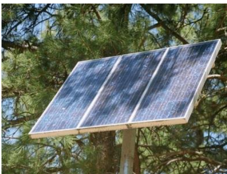
Figure 17 - Solar Panel with Partial Shade
